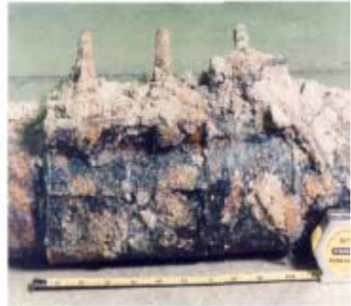
Two clamps on water main
